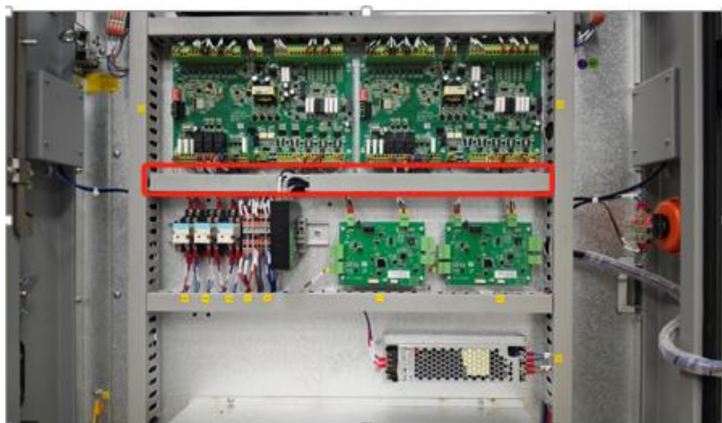
Figure 6-26 Location of Cable Dust Cover
